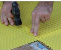
**3.3.-** Fix with double-sided seal, depending on model. A doublé-side seal applied on the perimeter of LHV formliner, and stripes is applied every 20/30, if required. Then, fix the LHV Formliner on the formwork panel.
