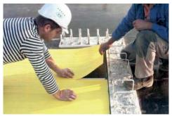
**4.-** Remove the LHV Formliner . This is done easily done; simply pull it from either end. In case of glue residue, can be used solvent or similar product to clean the formwork panel.
