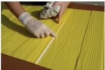
**5.-** Connect the sheets without sealing, knowing that the mark will remain in the concrete and the concrete could penetrate between the LHV Formliner and panel formwork.
